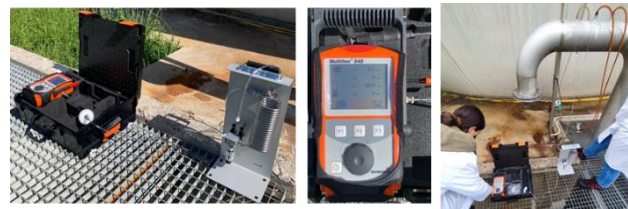
In situ hydrogen sulphide meter
